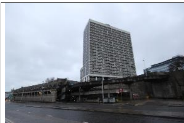
Type: Standard Title: Seamount Court, north elevation, above multi-storey car park, looking south. Alternative Text: Seamount Court, north elevation, above multi-storey car park, looking south, during daytime, with overcast sky, road to foreground. Date taken: 22/11/2018 Photographer: HES Copyright: © Historic Environment Scotland
